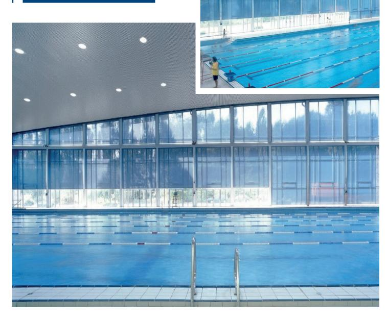
Standard roller blinds had already been discounted by the design team due to the sheer size of the glass façade. In practice, the film did not provide sufficient protection for the users, the heat and glare creating an uncomfortable environment.
