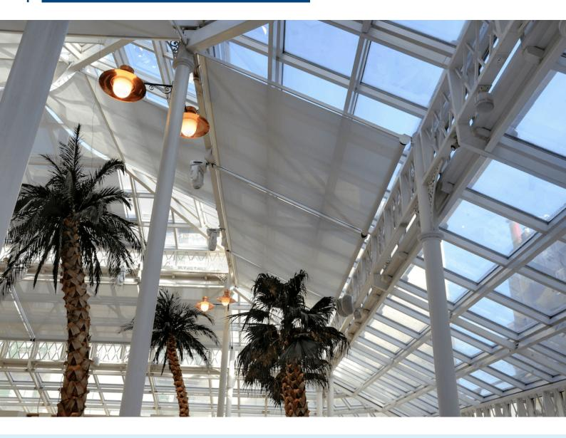
A single barrel mechanism keeps the fabric constantly under tension, and provides exceptionally smooth and quiet travel. We manufactured and supplied 16 systems of varying sizes, with the largest 4.125m wide.
