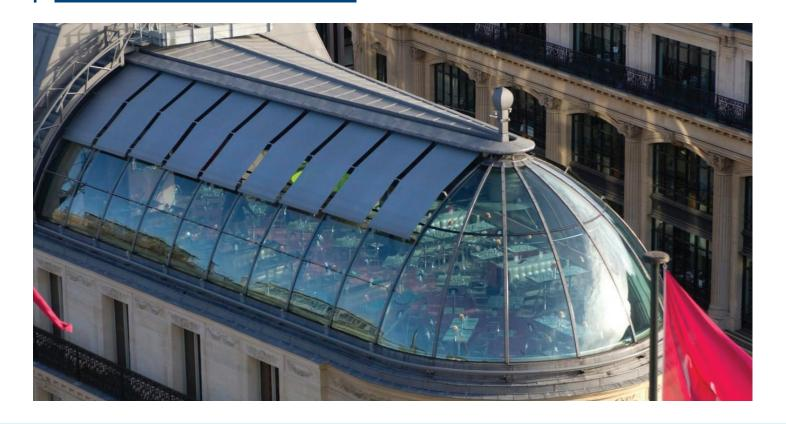
The TESS™ 420 system was selected for its strength and weather resistance, as well as its ability to minimise the load imposed on the structure. Retaining the tension force of the blind with its aluminium frame, it distributes weight evenly through multiple fixing points.
