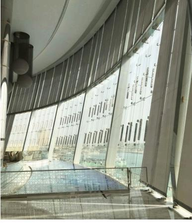
Architects DBI Design asked Levolux to design a shading solution for the large glazed façade in the lobby and special events areas. With a 15° incline and reaching 20m in height, each trapezoidal façade 'spine' was shaded using a single piece of fabric, fully retractable to reveal the stunning view when solar control was not needed, and translucent when deployed to allow a continued view to the outside.
