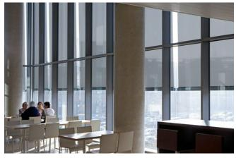
The interior included sloped parallelogram shaped windows in the restaurant area. Guthrie Douglas' engineers designed a bespoke zip tension system to follow the glazing mullions and maximise the internal floor plate, hiding the system mechanism within the ceiling void. The end result is a fully integrated shading solution which meets both performance requirements and aesthetic expectations.
