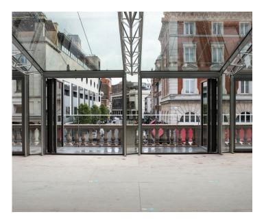
Guthrie Douglas worked with specialist Swiss metal façade contractor Tuchschmid to integrate external tension blinds into the roof structure, hiding a tensioned roller mechanism within the steel apex of the roof, and guiding the shading system along discrete stainless steel wire guides, almost invisible when the systems are retracted.
