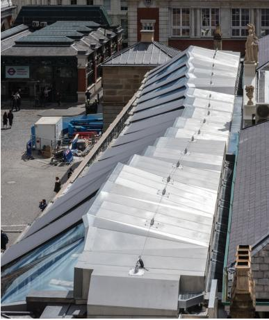
the design process to integrate bespoke shading systems that disappear into the surrounding structure when not in use."
