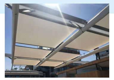
Each rooftop terrace required eight shading systems and in keeping with the light and airy feel of the buildings, they were each fitted with TESS™Poly 5% in white. Made from tear-resistant polyester, the material has a PVC coating with fungicidal and dirt-repellent finish and UV absorber. It is also flame resistant according to DIN 4102-B1.
