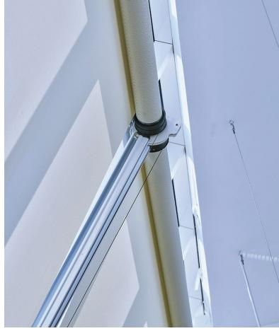
the tension force of the blind, and the weight of the system is distributed via multiple fixing points. This means that the systems could be fixed at the specified height leaving a section of glazing uncovered. Controlled via Somfy IO Oximo digital motors the tension blinds provide an easy to use solution, which creates an optimum working environment for the staff using the offices.
