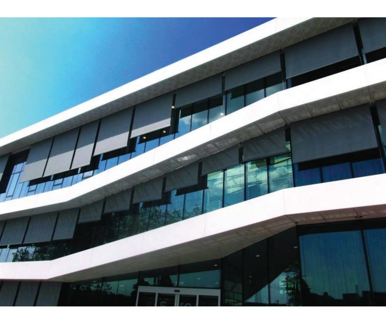
Boasting an almost entirely glazed façade the building design required an intelligent shading solution. The external façade benefits from a TESS™140 external blind system.
